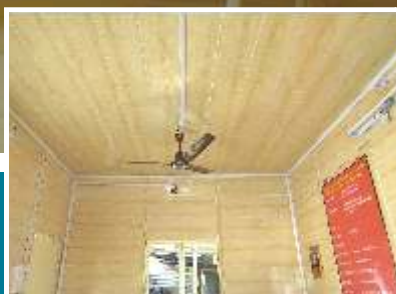
FALSE CEILING FOR OFFICE
